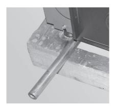
Fig. 10 Sliding the boiler off the pallet
