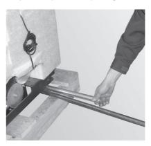
Fig. 9 Placing an iron rod under the boiler
