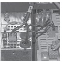
Fig. 101 Installing and connecting the frequency converters
