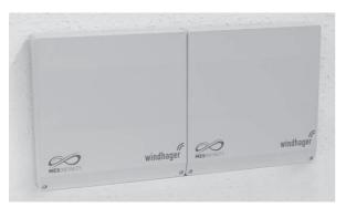
Fig. 137 Function modules (MES INFINITY control system) installed on the wall
