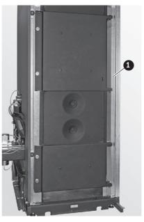
Fig. 43 Installing the cladding bracket 1.....Cladding bracket
